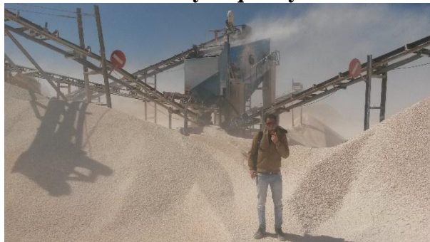
Fig. 7: Field image showing the third stage (i.e. production of aggregates) in the Al Abyar quarry.
