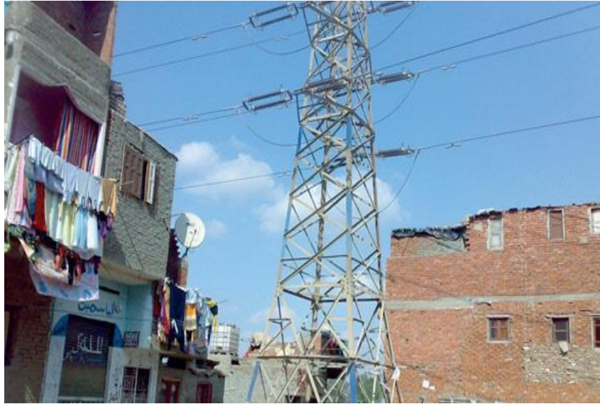
Fig (1.2) Building under overhead lines[8]
