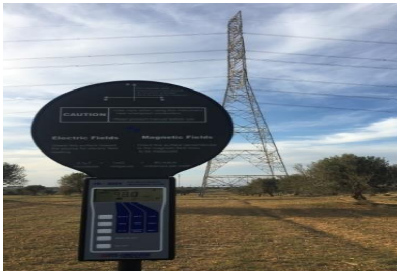
Fig (4.10) Electromagnetic meter survey
