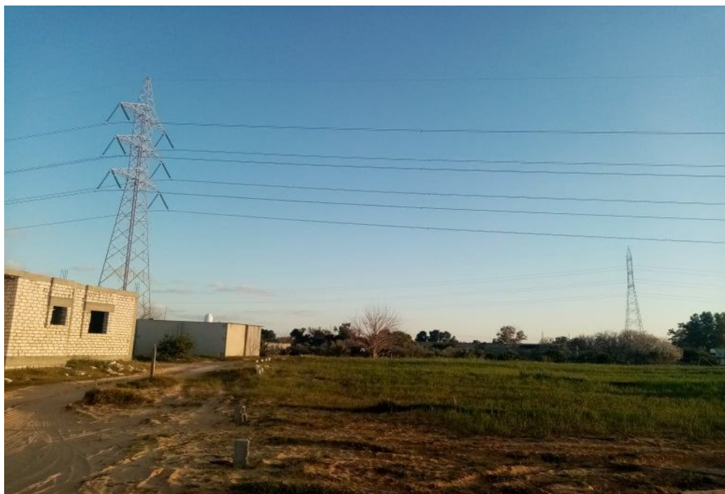
Figure(4-5) 220 KV voltage line that passes by a farm in the city of Zawia, Al- Barnawi area
